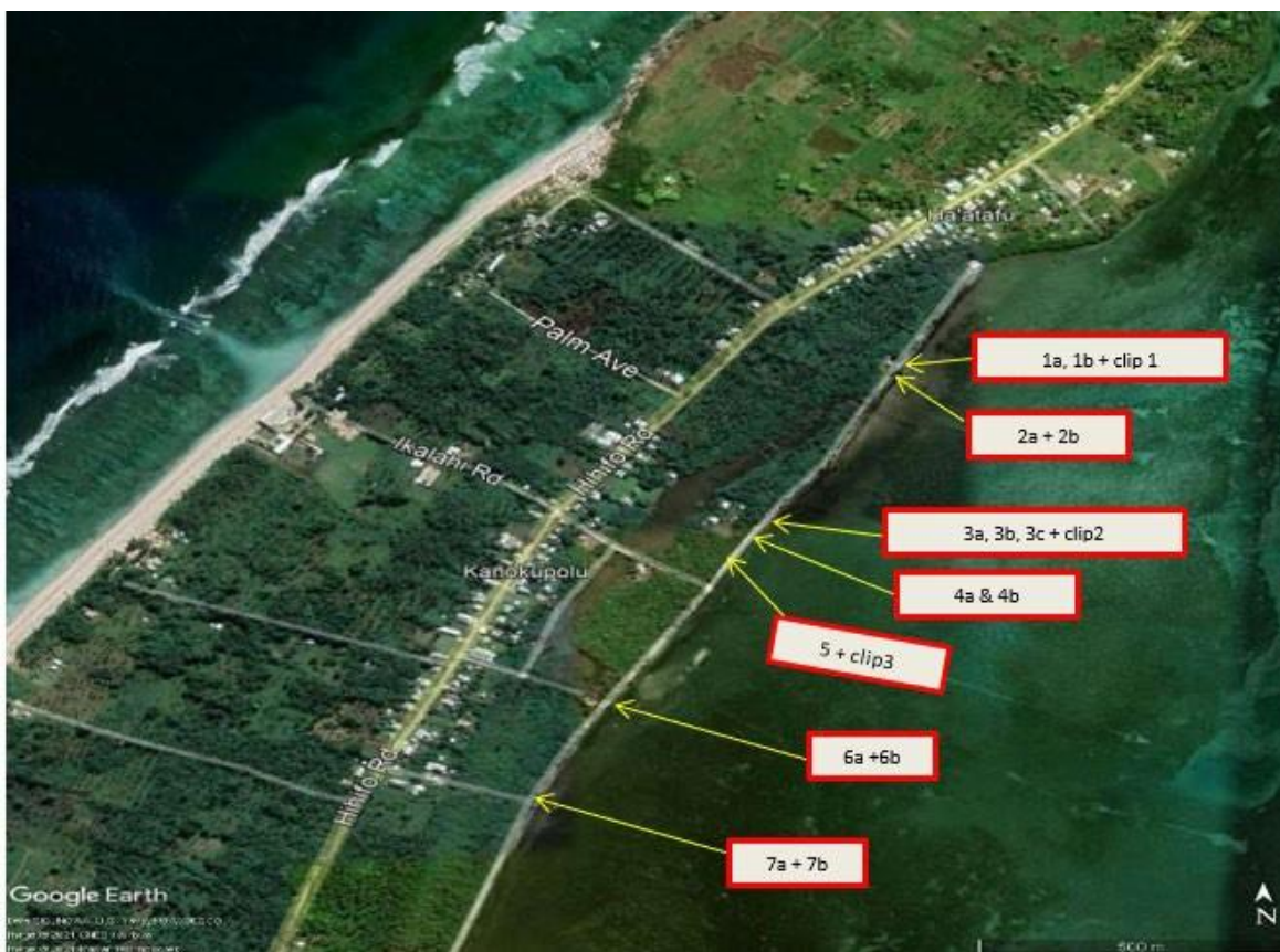
Sites of significant damage along the northern 1,350 m of the revetment
