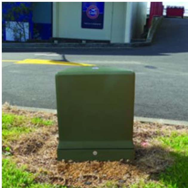
- Figure 24. Example of a pillar box. Source: Transnet
