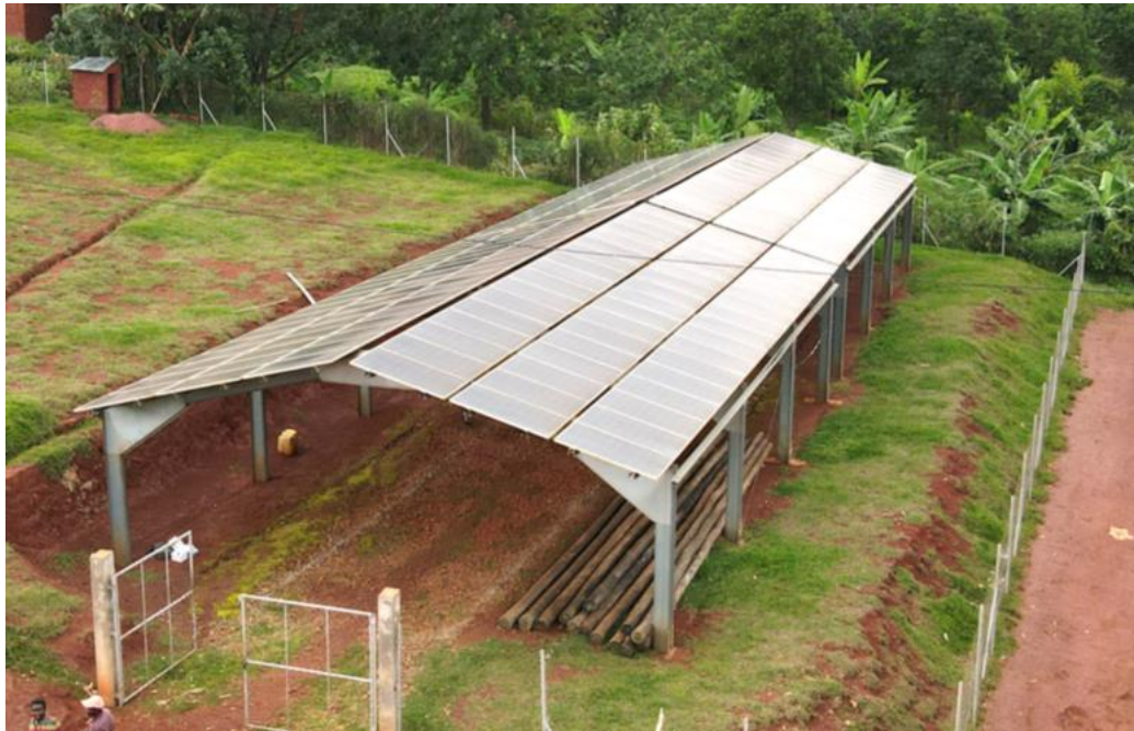
- Figure 13. Example of a 3m high canopy installation (those in Fefen will be waterproof). Source: TTA.
